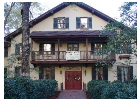
Retreat Center - main building.
